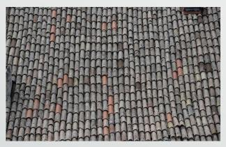
Partial subsidence or protrusion, severe loss of tiles: construction prohibited
