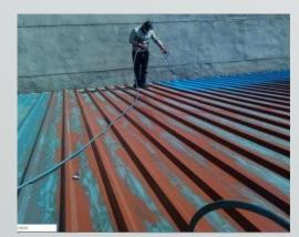
A large proportion of rust and stains found on the edge of cladded steel tile: construction prohibited
